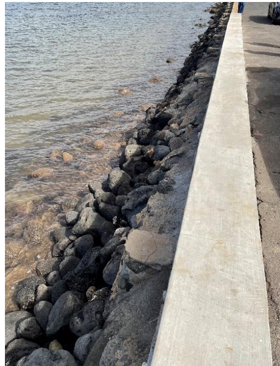
PHOTOGRAPH NO. 3: Example of existing revetment to be repaired.
